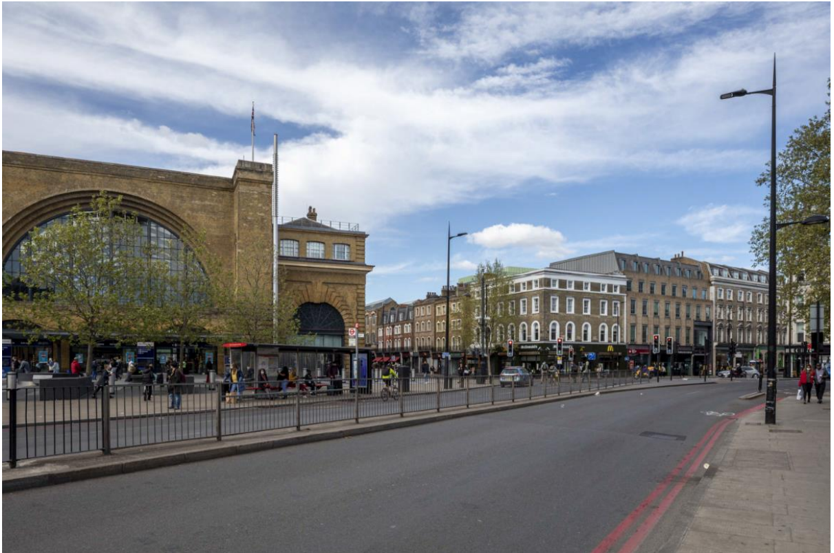
Image 40 – Rendered Verified View 13 from Euston Road towards the Site
