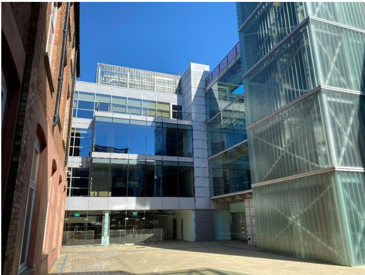
Image 8: Laundry Yard: Times House
