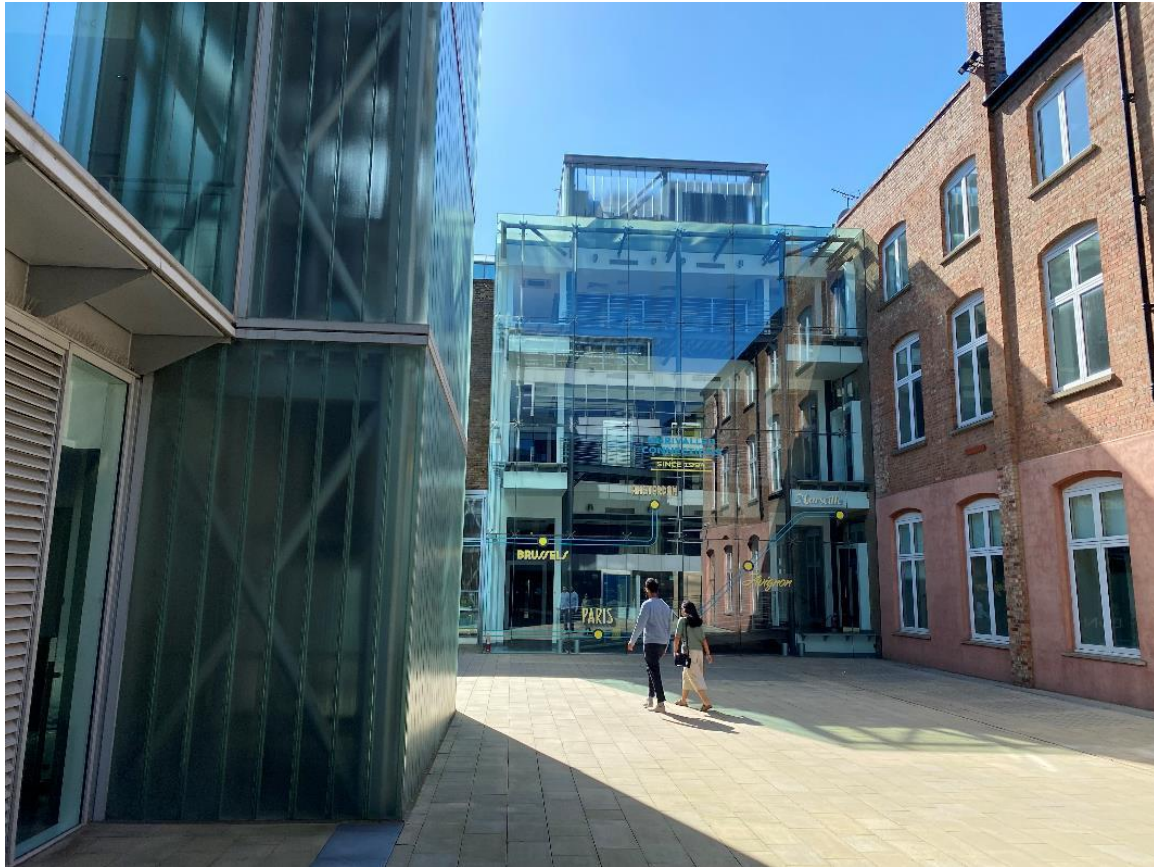
Image 7: Laundry Yard: Times House (left) and Laundry Building (right)
