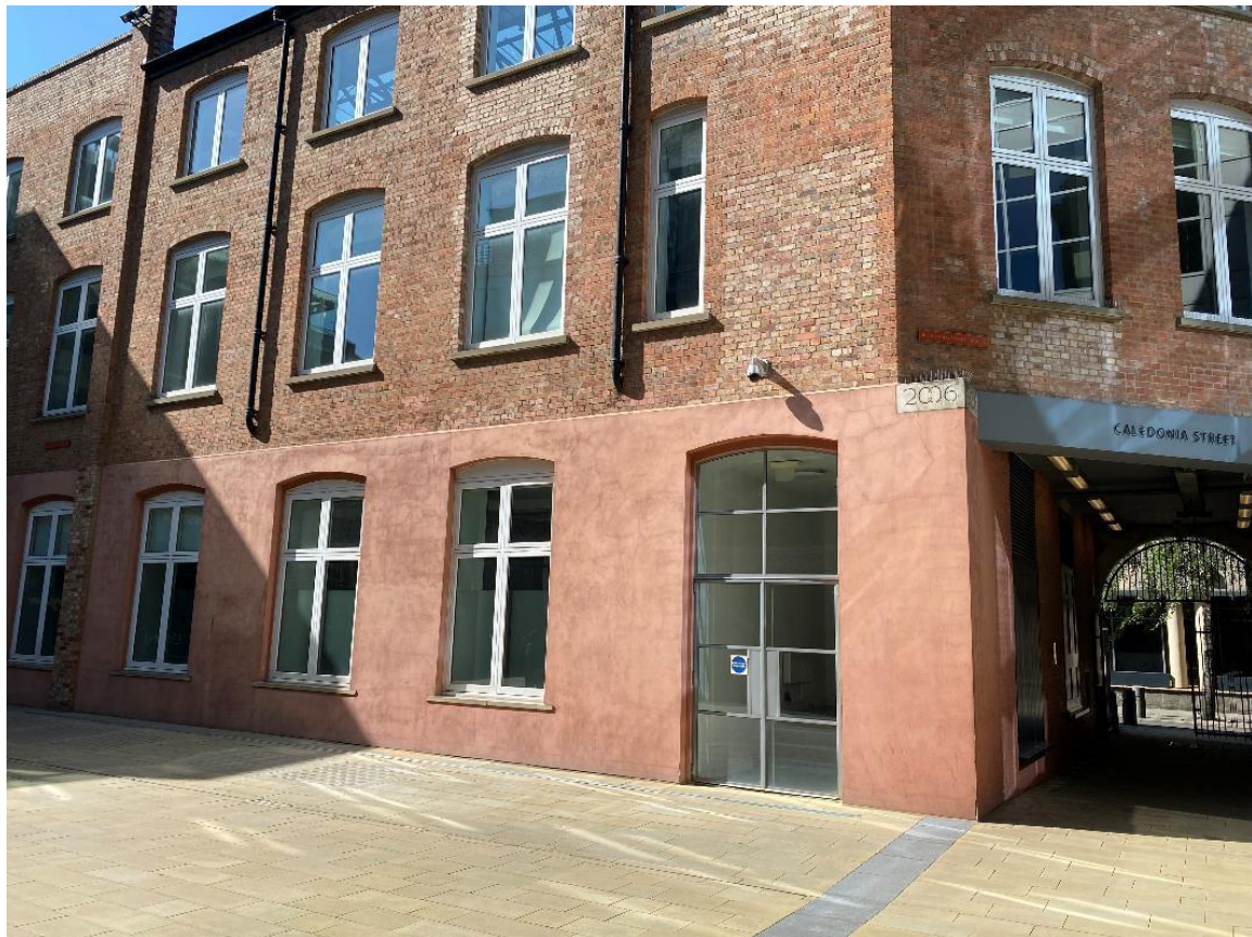
Image 6: Laundry Yard: Laundry Building
