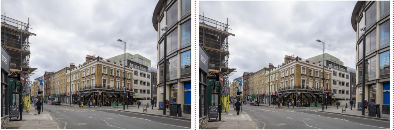
Image 37 – View 10 Comparison - As submitted Rendered Verified View 10 - View looking south east from Caledonian Road vs CGI of revised scheme
